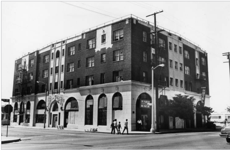
Exterior view of the Dunbar Hotel. The hotel is shown closed and in need of repair. Image made accessible through a grant from the John Randolph Haynes and Dora Haynes Foundation, Los Angeles Public Library.
