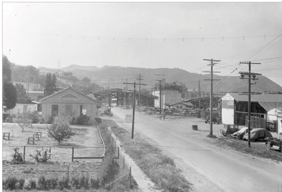
Construction of the Hyperion-Glendale Viaduct, looking towards bridge from Riverside Drive, showing houses in foreground and Griffith Park in background (ca. 1928) Collection of Los Angeles City Archives Department of Engineering Historical Photos
