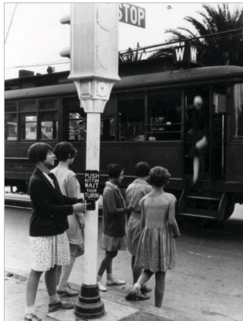
Pedestrian traffic signal
