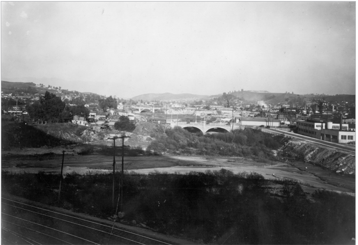
Construction of the Hyperion-Glendale Viaduct, looking towards bridge from Riverside Drive, showing houses in foreground and Griffith Park in background (ca. 1928) Collection of Los Angeles City Archives Department of Engineering Historical Photos
